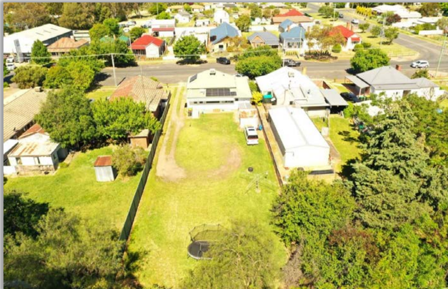
Drone View to East
